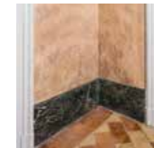
7 False wainscoting in the corridor
