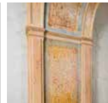
5 Faux marble in the eastern corridor
